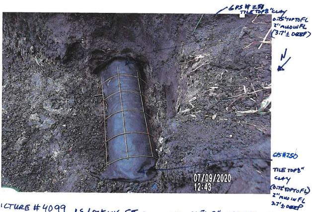
PICTURE # 4099 IS LOOKING SE SHOWING ZILF 8" OW HOPE PERF TILE INPLACE WITH ZID'X3ID' FABRIC & 1.5'XZID' G"X6"WIRE MESH OVER JOINTS BEFORE 3/4 CONCRETE COLLAR POURED
