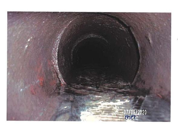
PICTURE# 4103 IS LOOKING UP STREAM INSIDE 8"CLAY TILE WITH ABOUT I" FLOW AT GPS #30Z (FOR 8"CLAY THE) (0.72' TOP TO FL)
