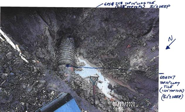
PICTURE# 4095 IS LOOKINGSE SHOWING Z.6 LF. PIECE OF 15'DOW HOPE NOWPERF THE IN PLACE FOR REPAIR WITH BEDDING ROCK UNDER TILE
