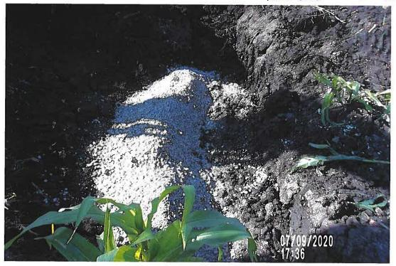
PILTURE# 4124 IS LOOKING NORTH WEST SIDE OF COHWYSZT SHOWING 4" HOPE PERF TILE REPAIR BEDDED WITHROCK.
