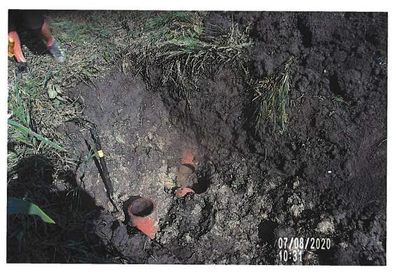
PICTURE# 4057 IS LOOKING NW SHOWING SECTION OF 8" CLAY TILE ROLLED OUT IN SOUTH DITCH OF COHWY DY! NW OF BEEHIVE INTAKE FOR CREW TO RUN LOCATOR CABLE UPSTREAM TO FIND PLUG IN TILE.
