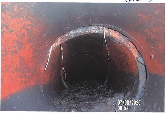
PICTURES 4052 IS LOOKING NW UPSTREAM INSIDE 8"CLAY TILE WITH Z"+ OF MUD IN FLOWLING FROM GAS# 250. TILE IS IN 6000 SHAPE WITH PEW FINE ROOTS AND A FEW OFFSET JOINTS
